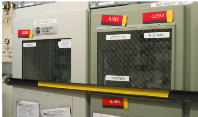
Figure 3. Process Gasses are closed
